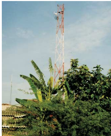
Touching base: transmitters connect corDECT users up to 25 kilometres away to the central unit.
